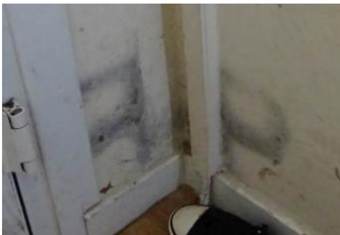
S17 – 12A Lawnside, Forest Green, Hall mould in square shapes on front & alleyway walls
