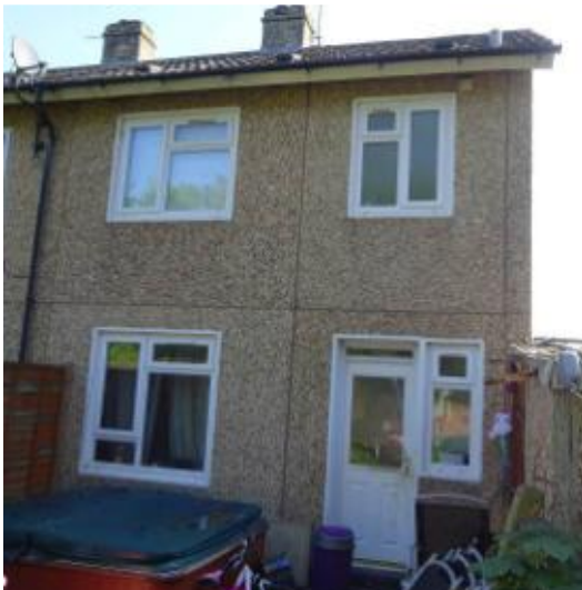
S3 – Typical Rear Elevation, semi-detached house A
