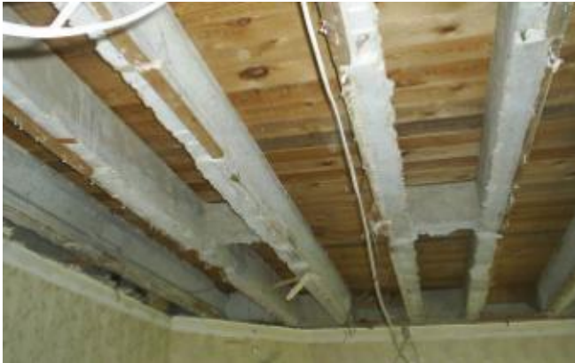
S49 – View of typical PRC "ladder" beams from below (not SDC stock photo)
