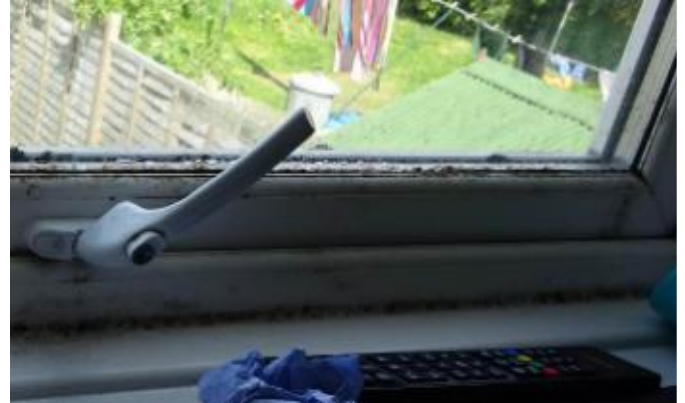
P8 – 14 Mosley Cresnet, Cashes Green, mould on window frame in rear bedroom
