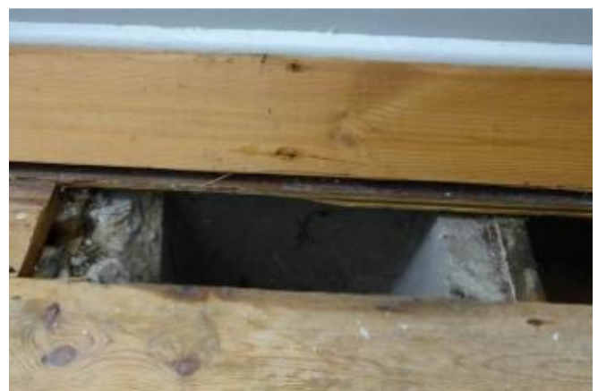
S48 – 6 Upper Park Road, Nailsworth. First floor construction, PRC ladder beams (see S49 for general view, taken in another house not in SDC stock)
