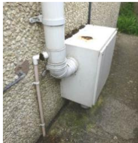
Q16 – Example of Radon Pump (to 1 No in Badgers Way, and 3 No in Woodpecker Way)
