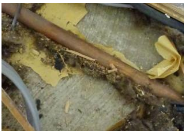
S47 – 3 Upper Park Road, Nailsworth. First floor, suspended cast in-situ concrete slab under floorboards and battens.
