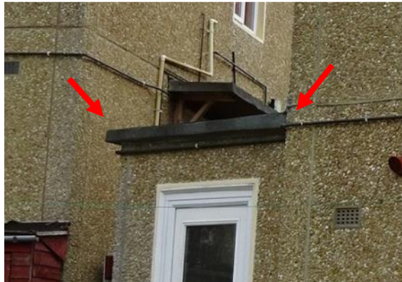
S55 – 5 Upper Park Road, Nailsworth. Flat roof side extension (compare with S39, lean-to roof No 6)
