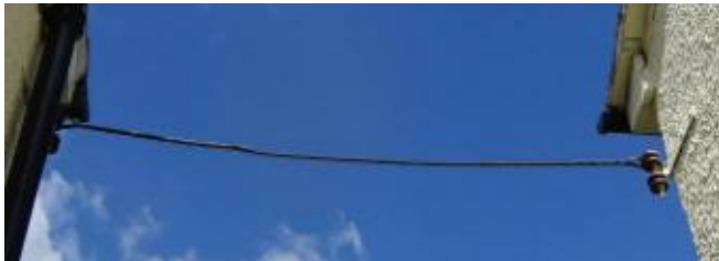
P9 – Typical overhead power supply cables between buildings (this one at 14 Mosley Cresnet, Cashes Green)
