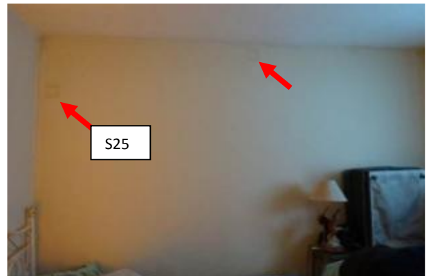
S24 – 45 Lawnside, Forest Green, bedroom gable wall, two small square areas of staining (arrowed). Photo S26 is to the right side.
