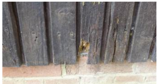
T24 – 6 The Knoll, Uley. Side, rot & woodworm to outer boards at dpc level
