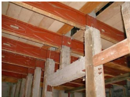
TYPICAL PARTY WALL Finishes removed showing columns
