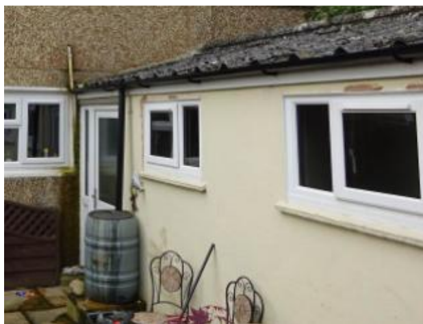
S59 – 26 Willow Road, Stonehouse. Outbuilding joined to the bungalow (note: Outbuilding is blockwork construction)
