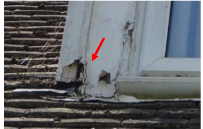
T36 – 3 Mount Pleasant, Wotton-Under-Edge. Rear dormer window poor paint finishes to framing & architrave
