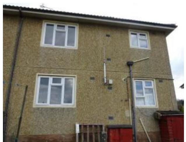
S12 – Typical Rear Elevation, flats
