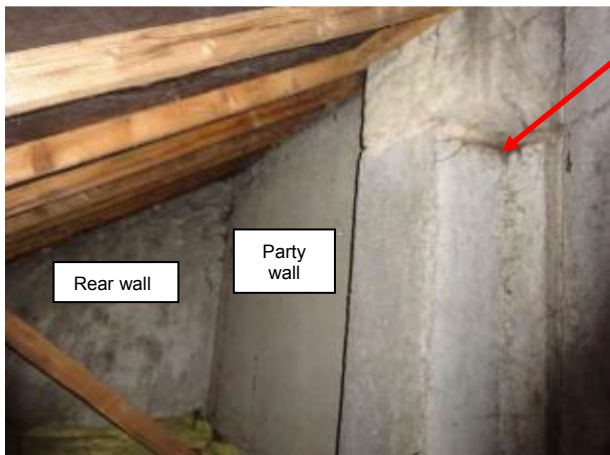
S53 – 6 Upper Park Road, Nailsworth. General view in loft towards rear & party wall
