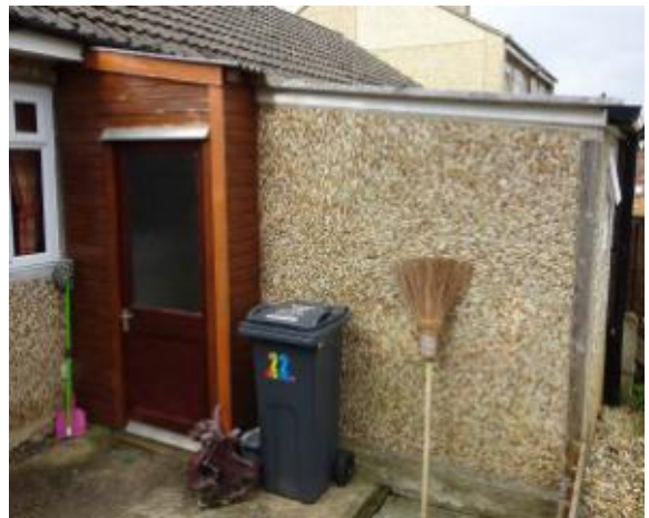
S58 – 22 Willow Road, Stonehouse. Outbuilding joined to the bungalow (note: Outbuilding is of Reema panel construction)
