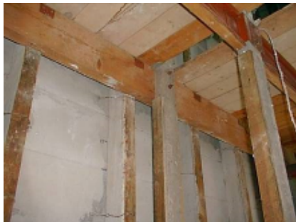
TYPICAL PARTY WALL Finishes removed showing columns
