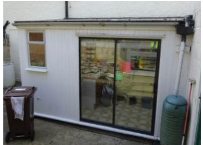
P4 – 14 Hyett Road, Cashes Green, Rear single storey extension
