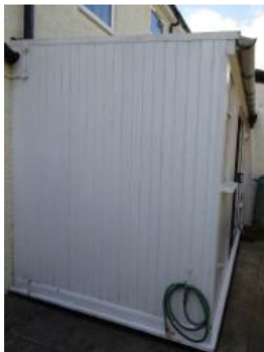
P5 – 14 Hyett Road, Cashes Green, Rear single storey extension
